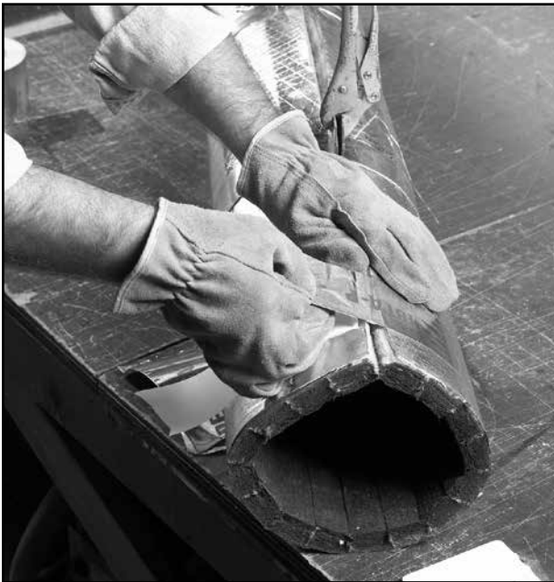
Figure 5-18. Applying crosstabs
