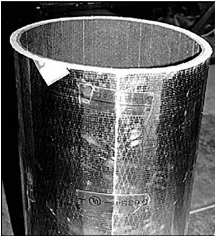
Figure 5-3. Joint taped
