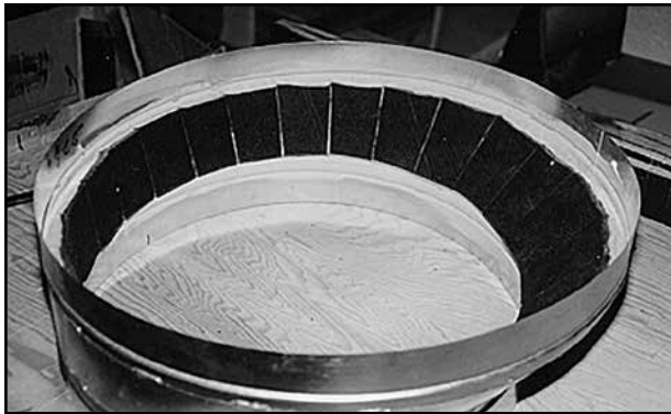
Figure 8-17. Tapered section installed
