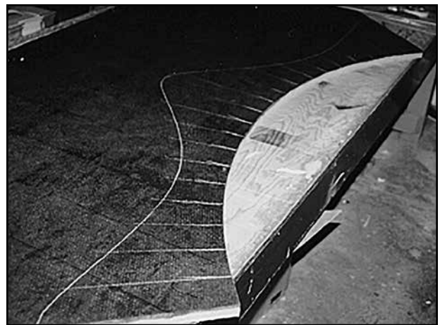
Figure 9-18. Partially cut fitting fab board
