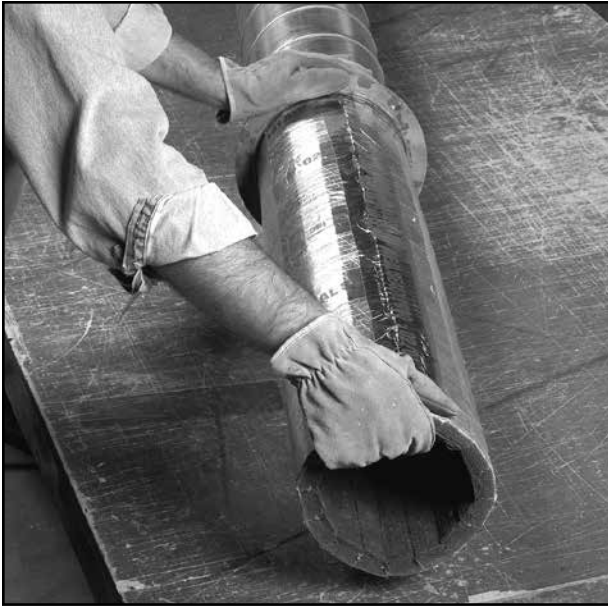
Figure 5-21. Slide insulation section into metal duct
