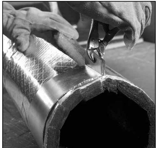
Figure 5-16. First drawband in place with clamp
