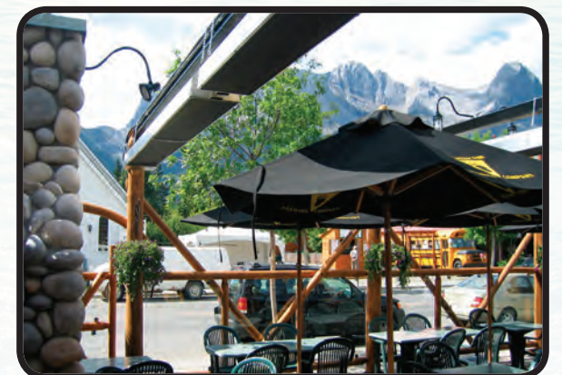
LOW CLEARANCE TO COMBUSTIBLES
